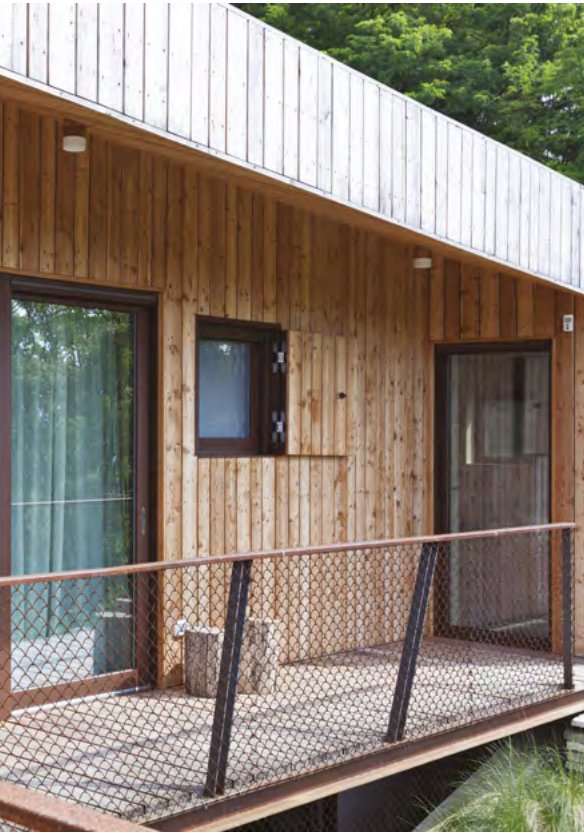
Outdoor installation of detectors
